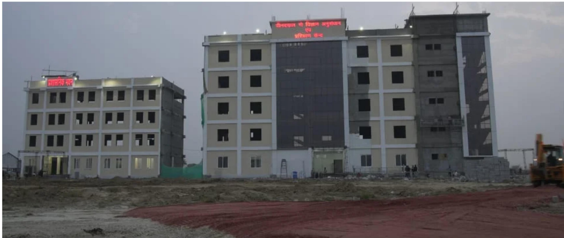
Construction site of Deendayal Cow Science, Research and Training Centre
