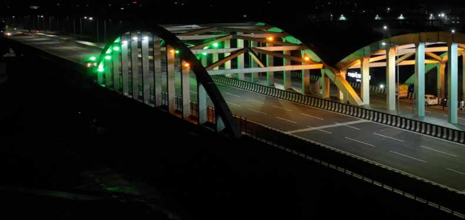
Aligarh-Kanpur Package-V Section of NH-91
